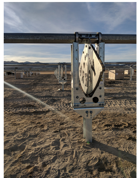
Photo (Right): Single-axis solar tracking at Railroad Valley Farms (Source: Railroad Valley Farms).
