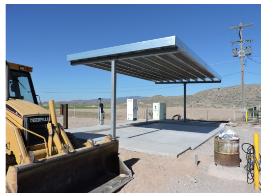
Photo (Right): Panaca EV charging station under construction (Source: Lincoln County Power District No. 1).
