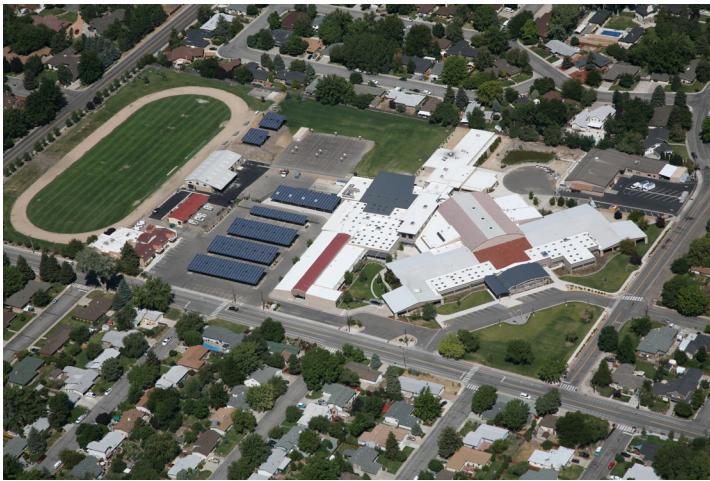
Photo: Solar Installation at Carson Middle School (Source: Carson City School District).
