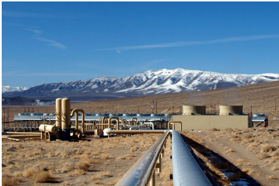
Photo: Ormat's Brady Geothermal Complex (Source: Ormat).
