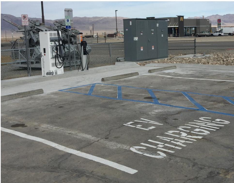
Photo (Left): Construction nearly complete at the Hawthorn EV charging station, which is part of the Nevada Electric Highway along U.S. 95 corridor (source: NDOT).
